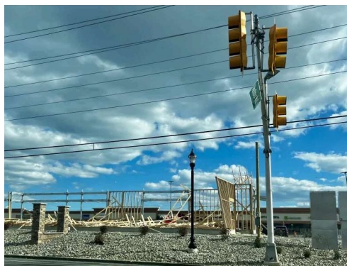
Wood framing is strewn about the Burger King construction site after heavy winds knocked them down. Hurricane clips hang on the remaining foundation after the storm. Photo credit: Isaac Linsk.
